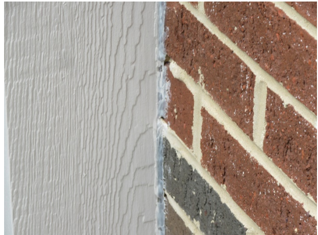
Overview of trim to masonry sealant
