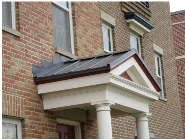
Metal roof overview
