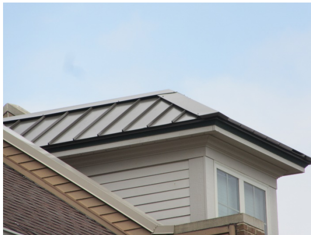
Alternate roof overview
