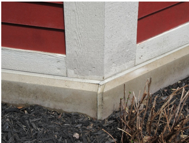
Repair at Unit 52
