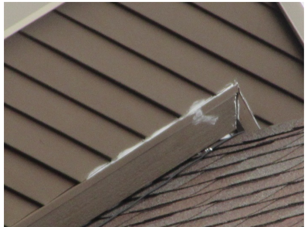
Discoloration at Unit 94
