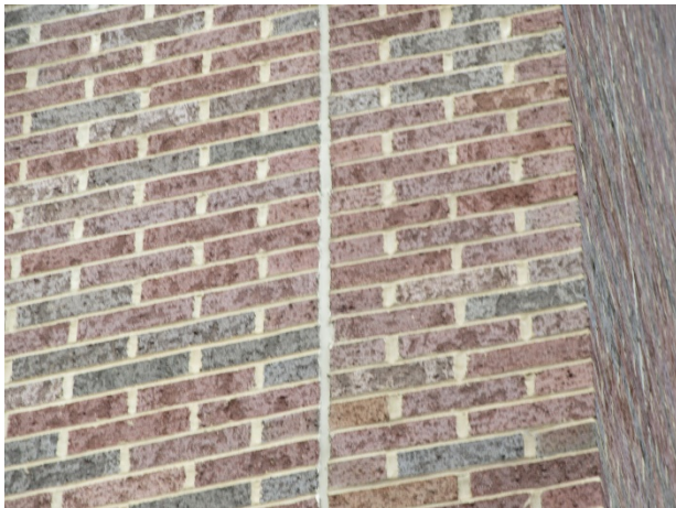
Control joint sealant in good condition
