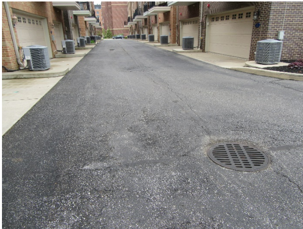
Overview of access drive between Buildings 1, 2 and 3
