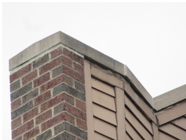
Coping overhang and sealant repair at Unit 21
