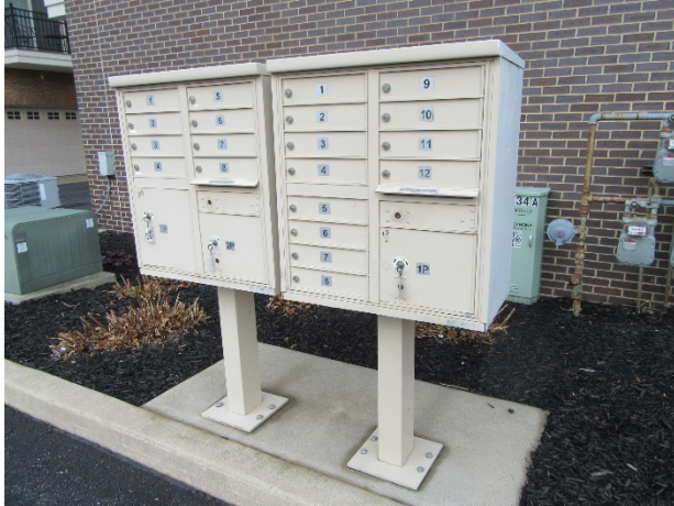
Mailbox station overview
