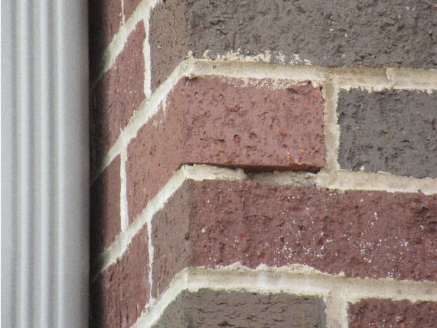
Mortar loss
