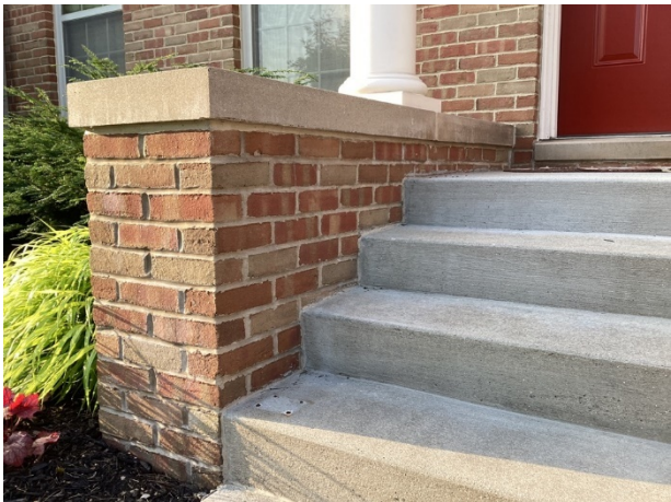
Wing wall overview
