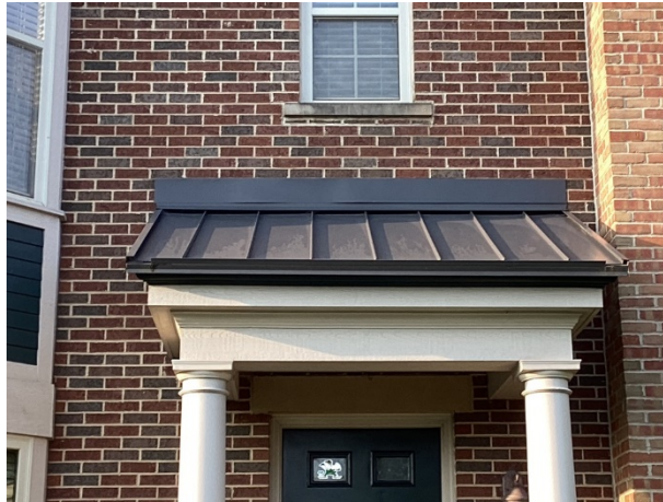
Metal roof overview
