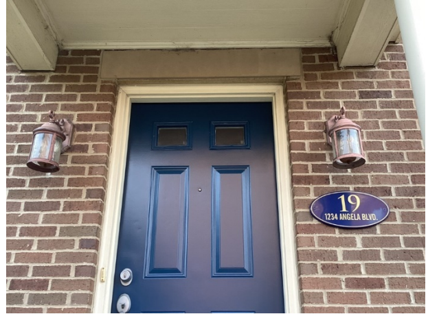
Wall mounted light fixtures at front entryway
