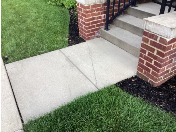
Sidewalk cracks
