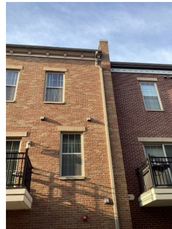
Building 1 gutter and downspouts overview
