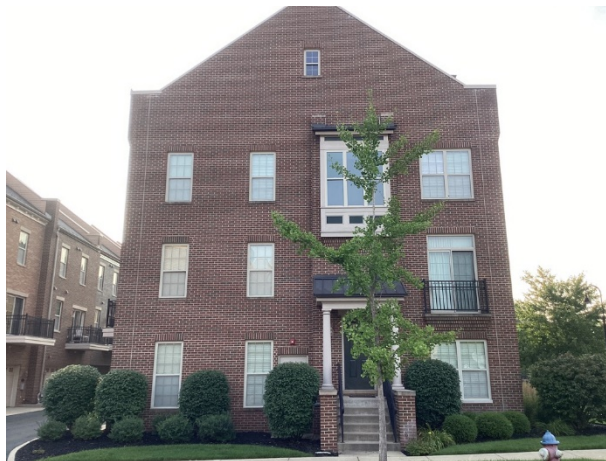
Side elevation overview
