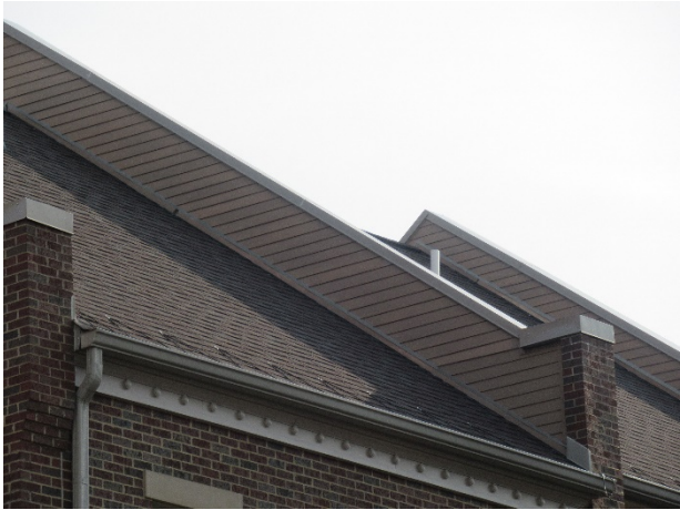
Parapet walls overview
