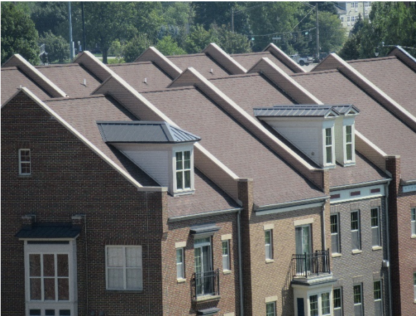
Asphalt shingle roof overview of Building 5
