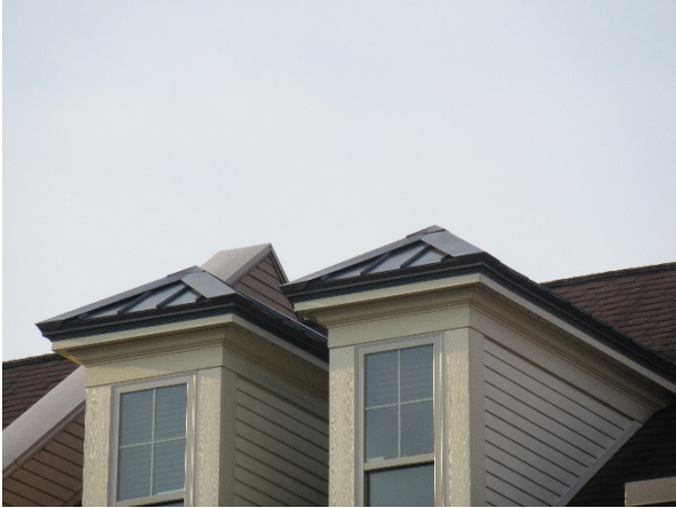
Metal roofs overview
