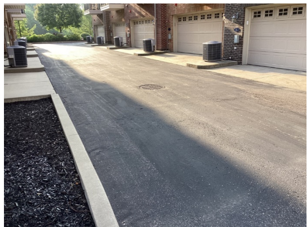
Asphalt pavement alley overview
