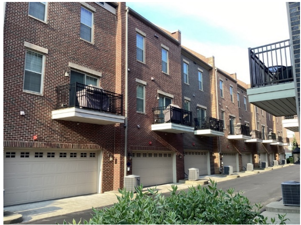
Rear elevation overview
