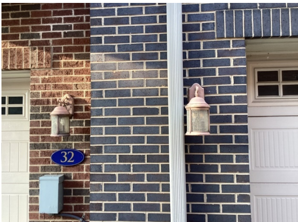
Wall mounted light fixtures at garages
