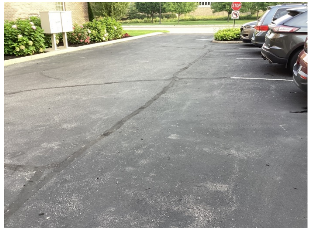
Asphalt pavement alley overview
