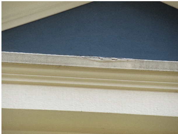
Finish deterioration
