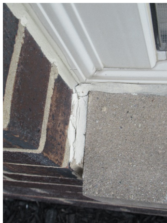
Sealant cracks
